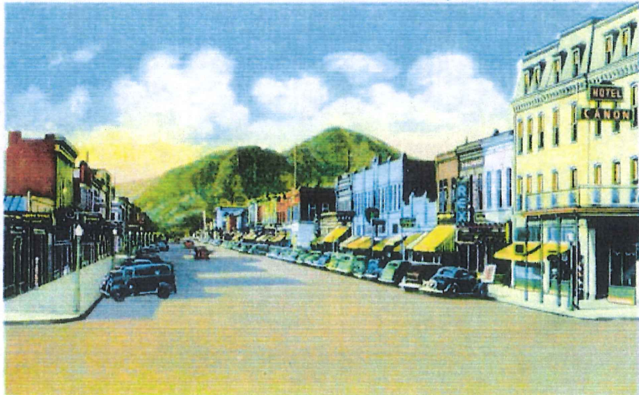
On U. S. 50, Transcontinental Highway at the Entrance of the Royal Gorge
